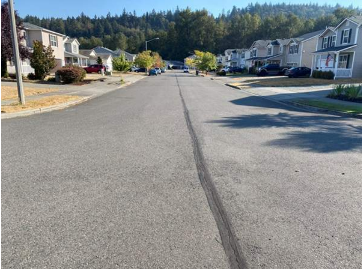
Figure 33. Crack Seal down Silvernail Street
