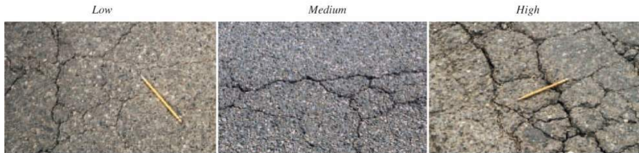
Figure 8. Alligator Cracking Severities
