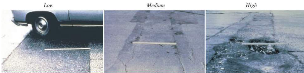
Figure 26. Patching Severities
