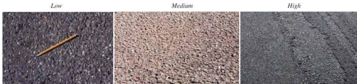
Figure 20. Raveling and Aging Severities
